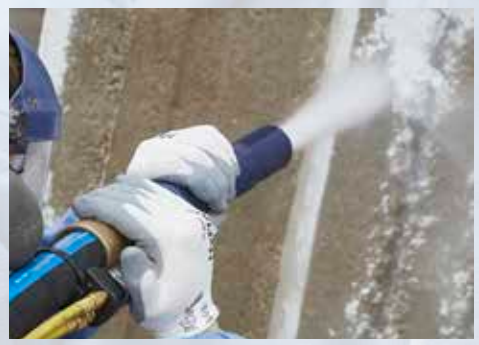
Concrete Surface Preparation
