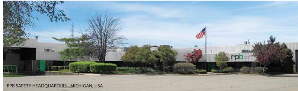
RPB SAFETY HEADQUARTERS - MICHIGAN, USA
