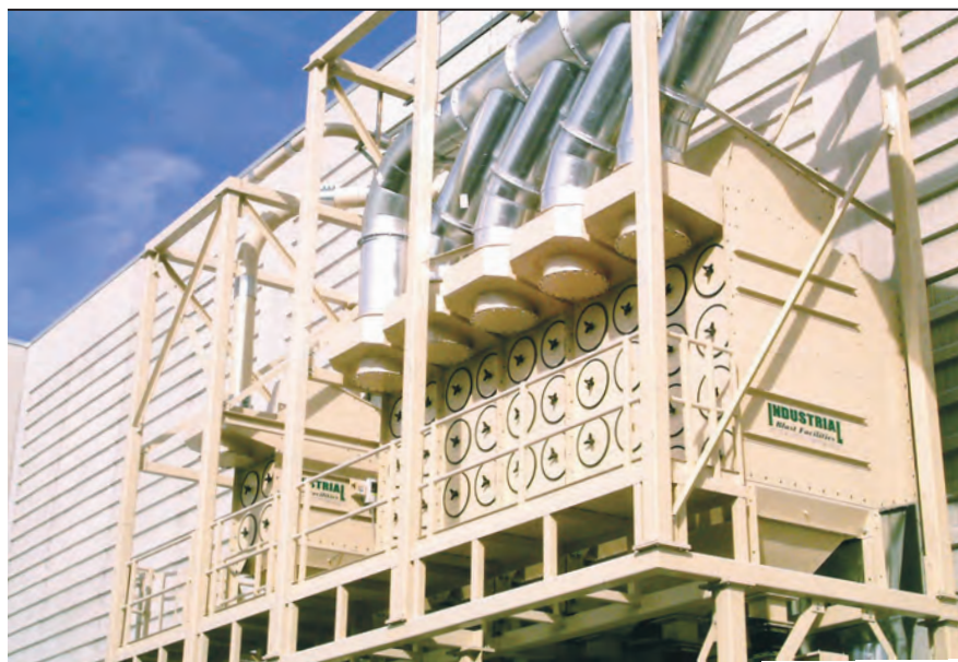
Two CDF's installed side by side at Hill AFB provide ventilation for both the recovery system and the blast room. CDF-8 on left; CDF-40 on right. Auger system transports dust to central collection area for disposal.
