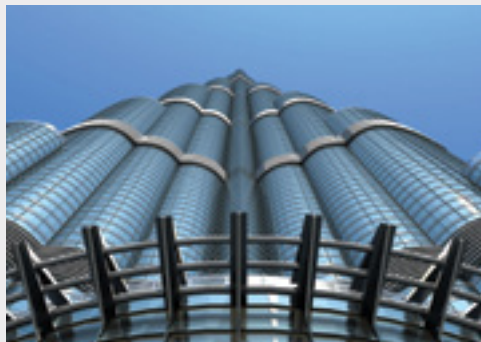
Burj Khalifa, Dubai, United Arab Emirates - The structural steel facets and frames were manufactured with waterjet machines cutting with GMA Garnet™.
